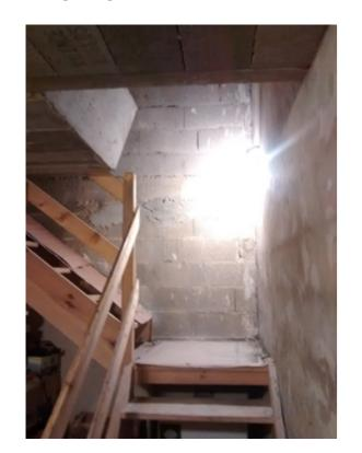
Plaster render on inner face of staircase walls for airtightness.
