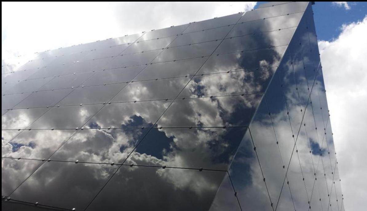
Photovoltaic ventilated facade
