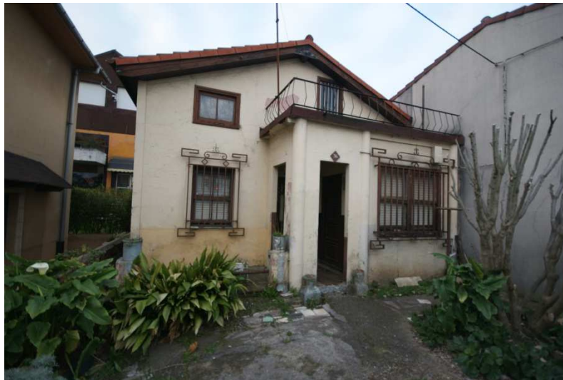
Figure 4: External view of the existing building. Front façade.
