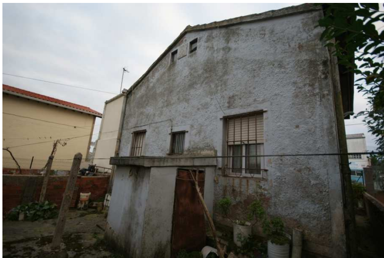
Figure 5: External view of the existing building. Back façade.
