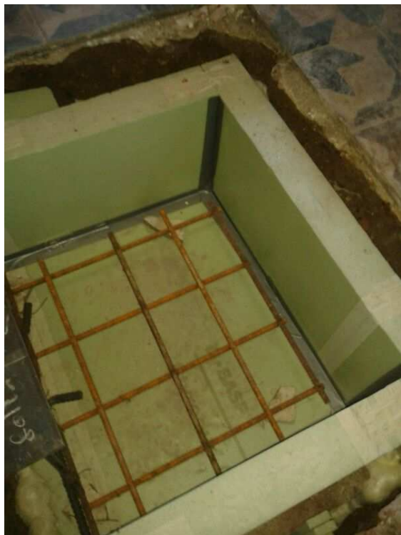
Figure 17: Insulation under the foundation
