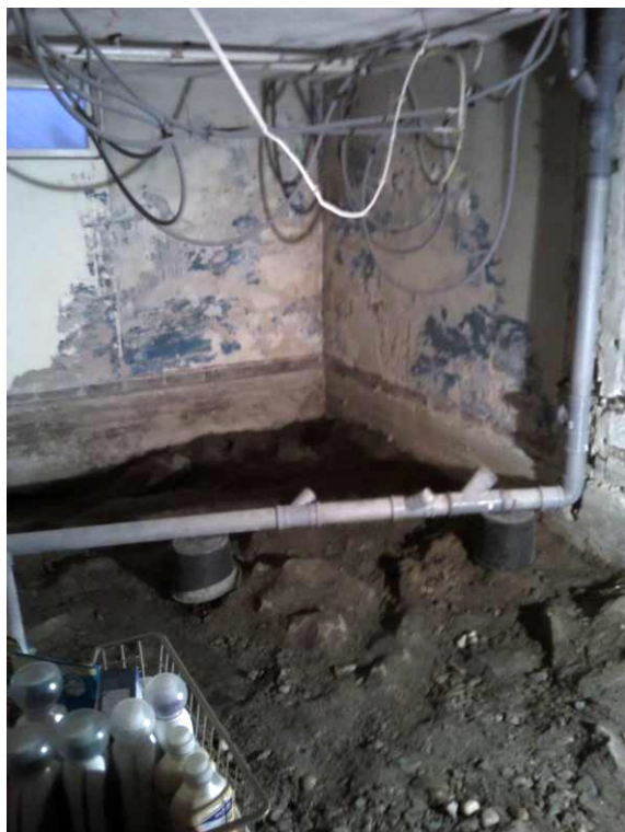
Figure 4: Lower floor dug up/concrete removed
