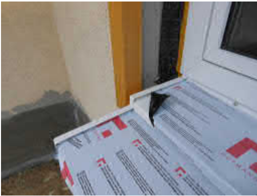
Existing window during the retrofit, before the thermal insulation has been installed: The timber frame in the insulation layer is required to fix the new window frame to it in future. The external, lower window sill will then remain, the second window sill will be removed. (Photo: Architect's office Werner Haase)
