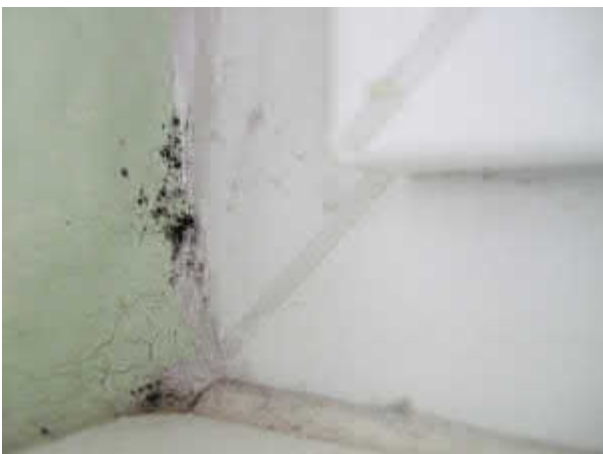
Figure 1: Onset of mould growth at the connection point of a window and an uninsulated wall
