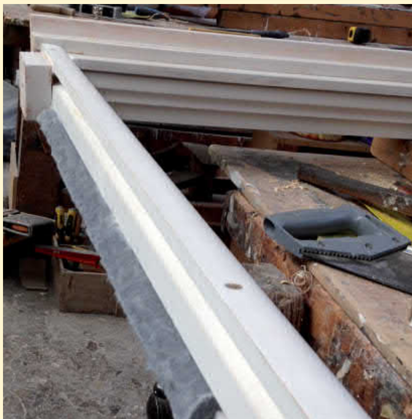
Figure 1 and 2: Construction sites of EuroPHit case studies in France Photo 1: Pollet Ingénierie Photo 2: Tillieux Menuiseries
