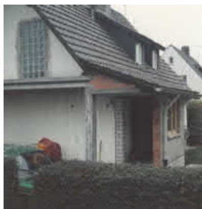
Figure 4: Additions to the original design. Entrance porch. Source: Karl Theumer
