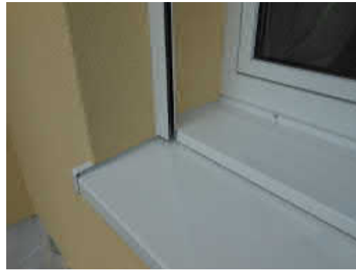
Interim solution with EIFC: Also the external blind is installed in the insulation layer. This way, it can remain even after the future installation of new windows and no works are required from the outside of the building. (Photo: Architect's office Werner Haase)
