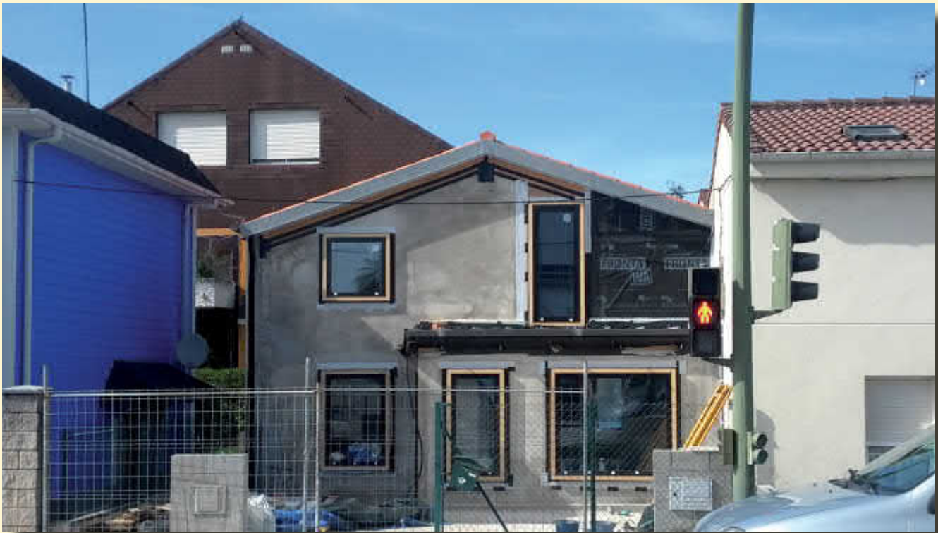
Figure 3: EuroPHit case study project „Centon“ underway in Spain, Photo: VAND arquitectura
