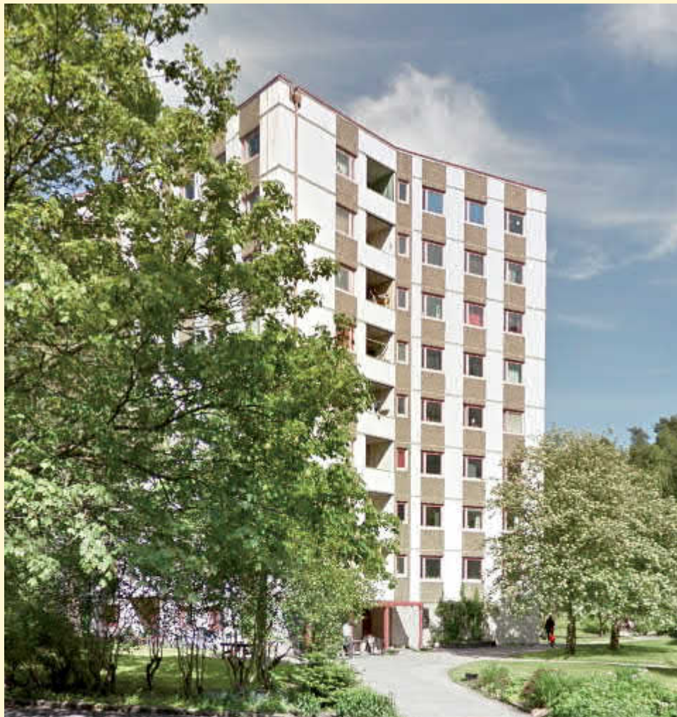
Figure 4: EuroPHit case study project „Gothenburg Stacken”, Sweden, before retrofit.
