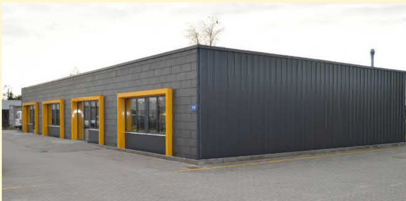
Figure 7 and 8: EuroPHit case study project „Rehab Workshop“ in Naesved, Denmark, before and after retrofit
