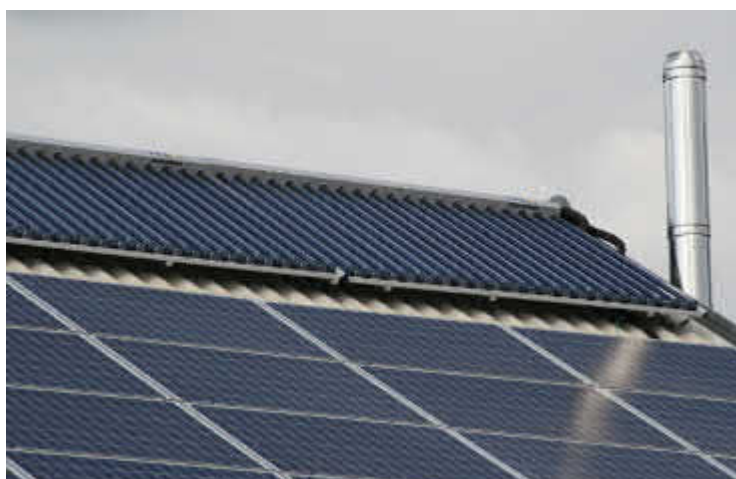
Figure 2: Example of a roof with solar installations
