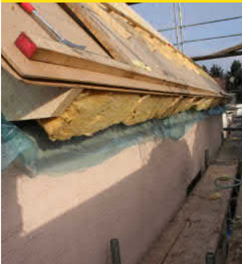
Figure 3: Roof edge with insulation above rafters – the airtight- ness membrane still has to be connected to the exterior wall.
