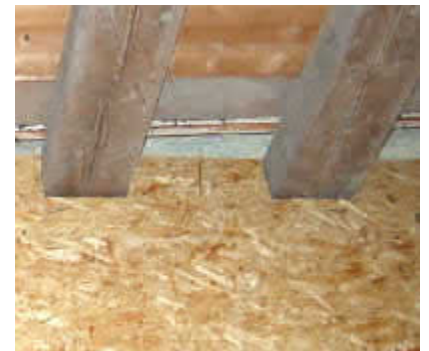
Airtightness (e.g. penetrations by beams)
