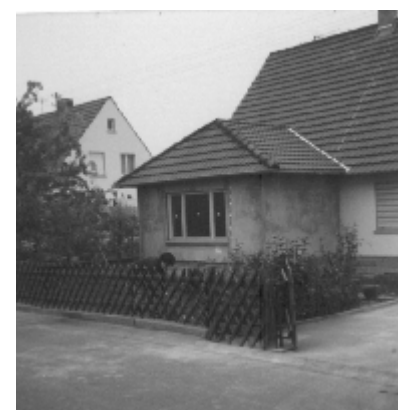
Figure 5: Additions to the original design. Living room extension. Source: Karl Theumer
