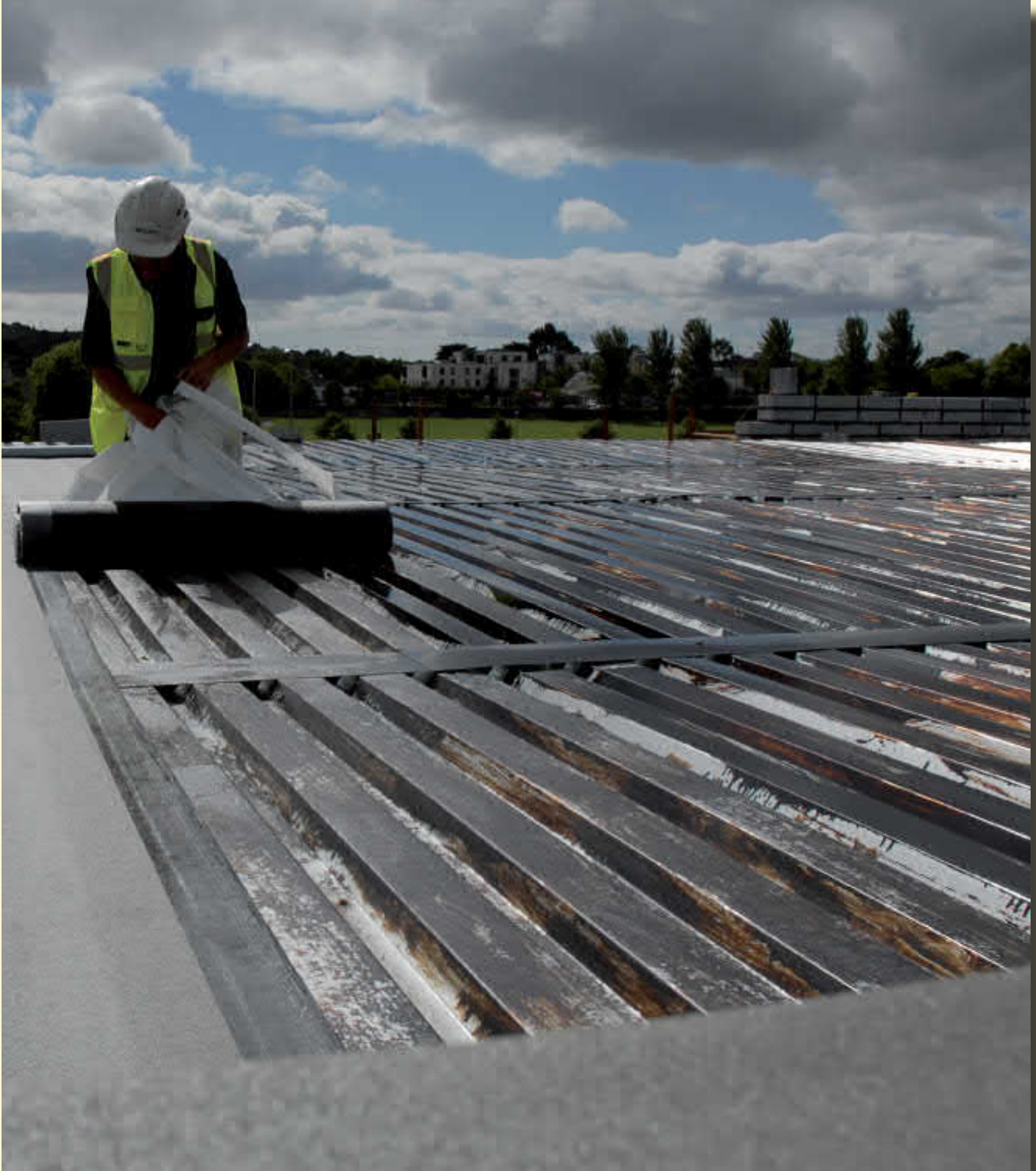
Figure 3: EuroPHit case study project „Home for Elderly“ in Dún Laoghaire, Ireland View of airtight layer being applied on new roof metal deck (Photo: Mariana Moreira)
