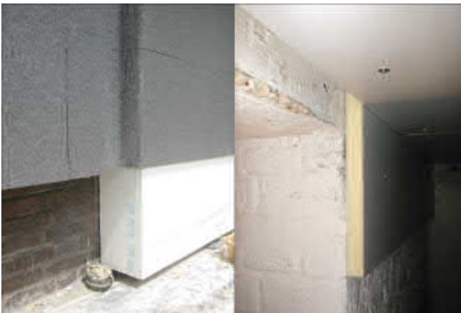
Figure 2: Connection of the basement wall to the basement ceiling: continuing the exterior wall insulation down to and well below the basement ceiling connection, and flanking insulation on the inside of the exterior wall of the basement mitigates the thermal bridge and provides for sufficiently high interior surface temperatures in order to safely prevent mould growth on the ground floor.
