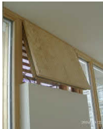
Figure 1 and 2: The most important means of passive cooling are movable shading and night ventilation
