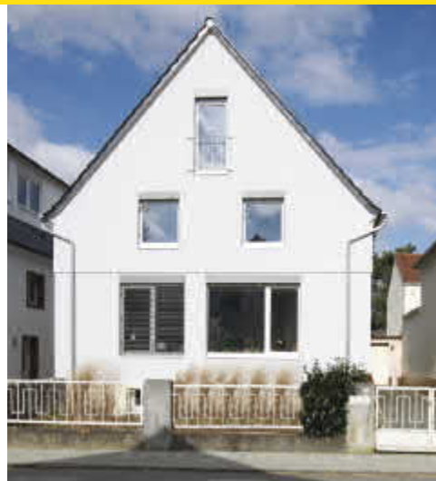
Figure 2: Single family home after a complete retrofit
