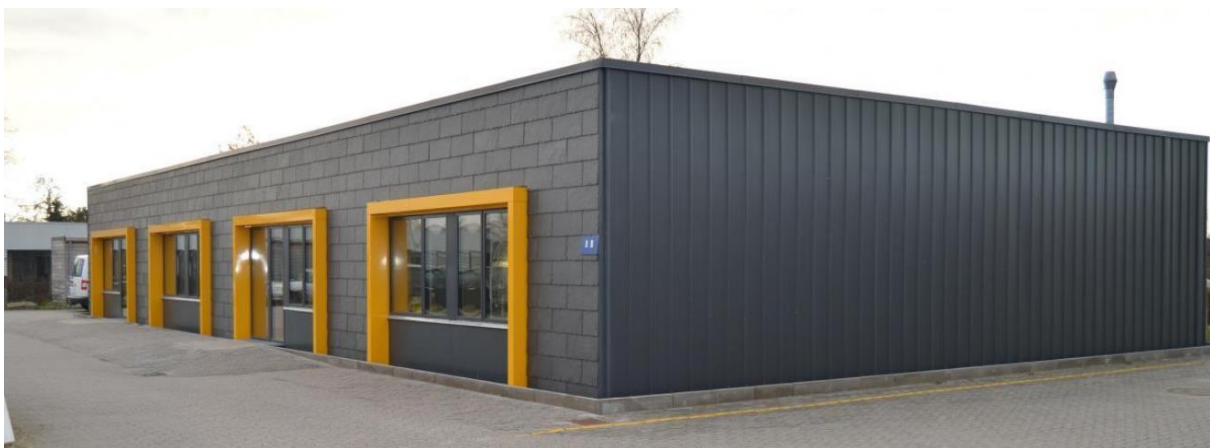
EuroPHit_CS13_Tommerupvej 8B_before retrofit (above), after retrofit (below) © Passivhus.dk
